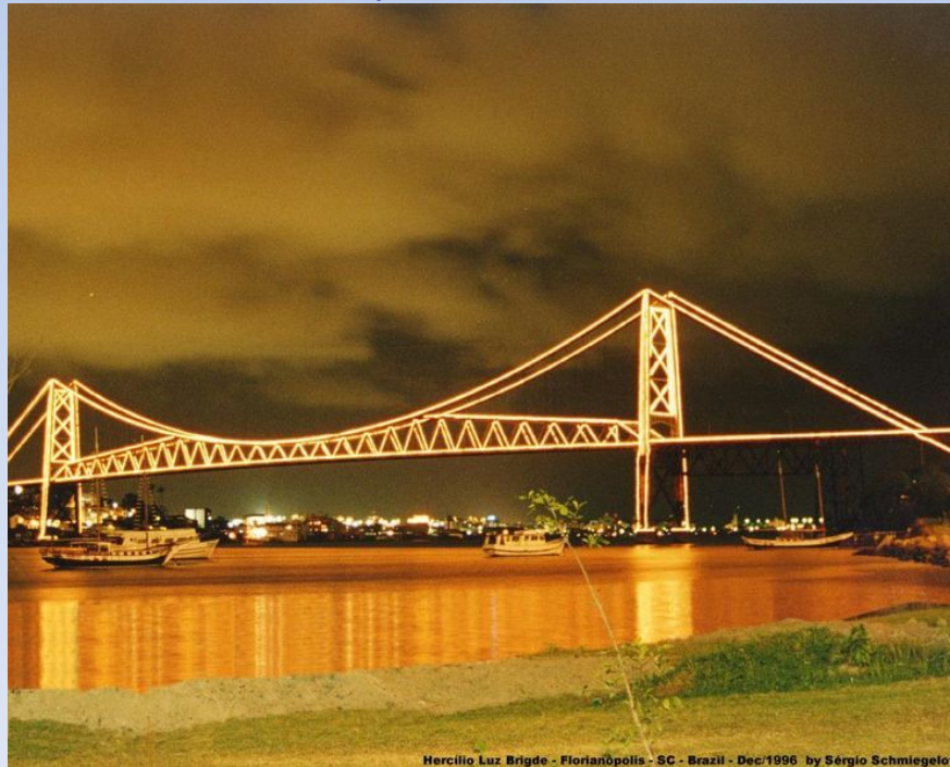
Hercílio Luz Bridge - Florianópolis - SC - Brazil - Dec/1996 by Sérgio Schmiegelow
